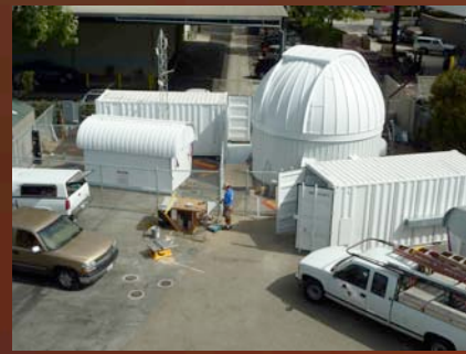
June 2010: Back Parking Lot (BPL) site in Goleta. Aqawan clamshell for up to two 0.4m, Weather, Dome for 1m, site-services building (SSB) container. The SSB and Aqawan in right foreground are for CTIO. See 7737-24 for Site Development.
