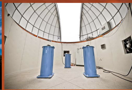
Piers waiting inside the modified Ash dome. Dome shutter control panel, fans and 1m control panel. Dome has 2m-wide shutter opening.
